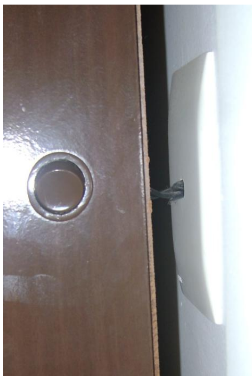
Figura 24 – Interruptor inadequado
