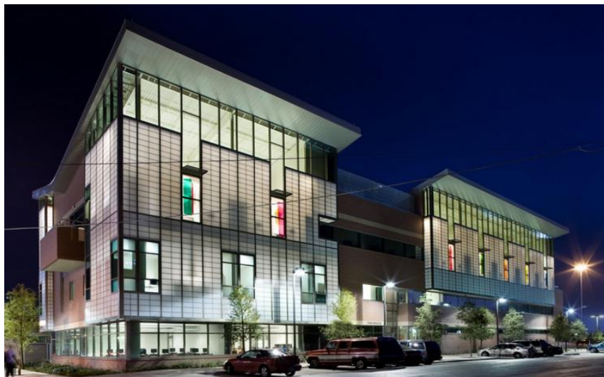
Figura 11: The Bridge - Vista Fachada
