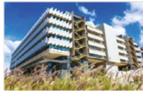
Siemens Middle East HQ LEED Platinum and 3 Pearl Estidama certifications. MEEED Quality Award for Projects 2013.
