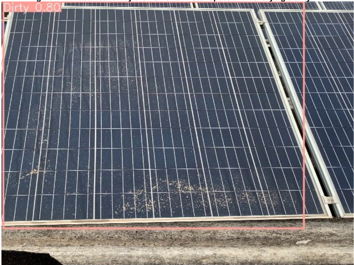
Figure 51 - Classification by the YOLO for visual spectrum identifying a dirty PV.
