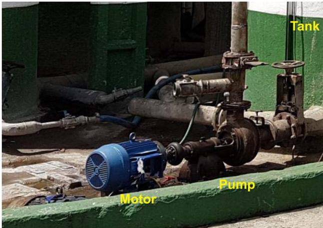
Fig. 3. Experimental setup in field with pump and motor used for water treatment.
