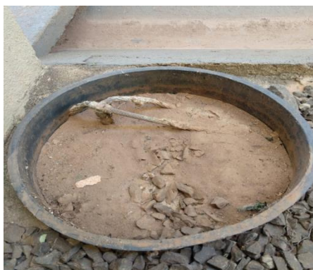
Figura 36: Descida 5 (Bloco P).
