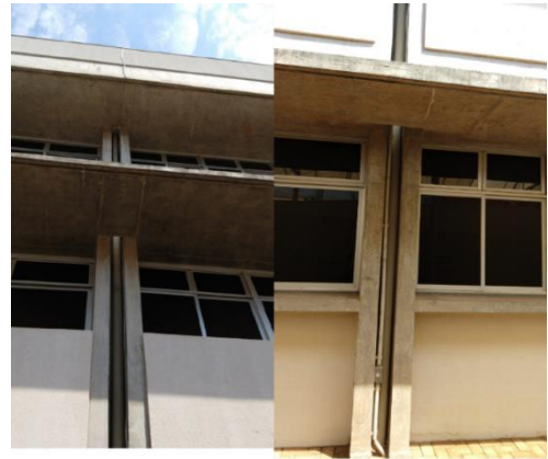
Figura 21: Descida 2 (Bloco P).
