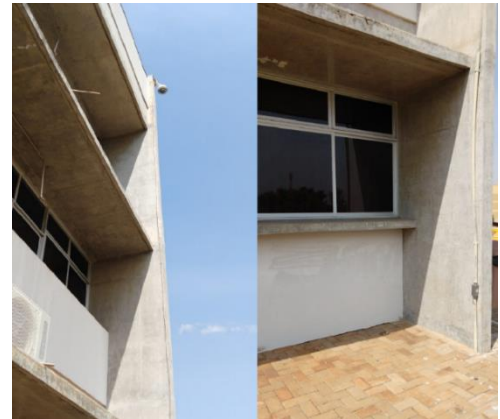
Figura 29: Descida 10 (Bloco P).
