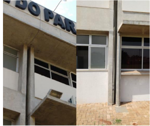
Figura 27: Descida 8 (Bloco P).
