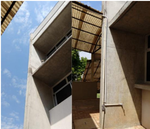
Figura 20: Descida 1 (Bloco P).
