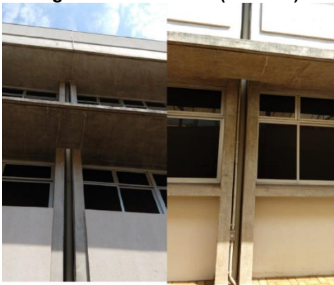
Figura 22: Descida 3 (Bloco P).
