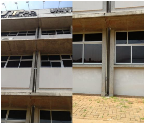
Figura 28: Descida 9 (Bloco P).
