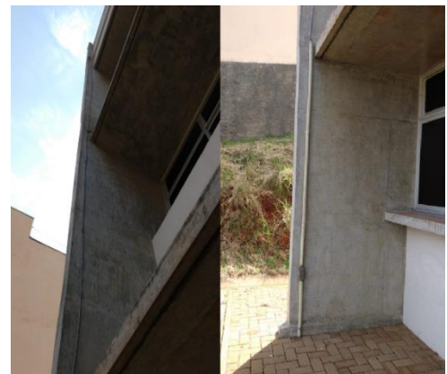
Figura 25: Descida 6 (Bloco P).
