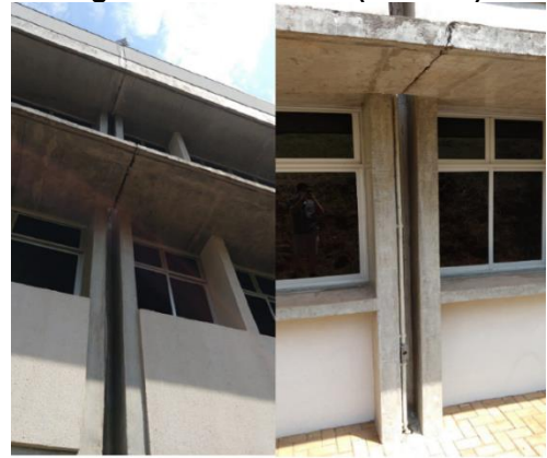
Figura 23: Descida 4 (Bloco P).
