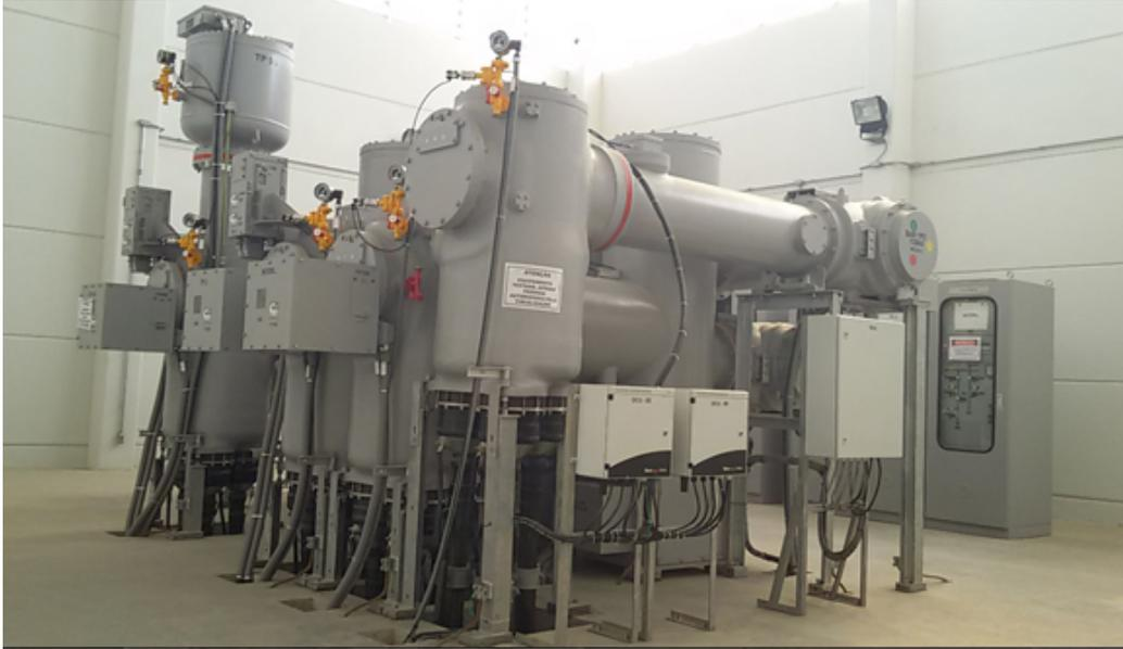
**Figura 13 – GIS (Gas Insulated Substation).**
