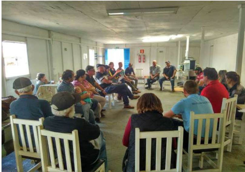
Photo 4 - Group meeting at the dam construction site, 11th of June 2018. Image source: the author.
