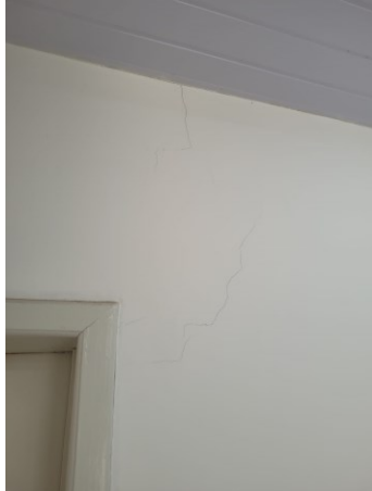
Figura 25 – Recalque (Fi=3)
