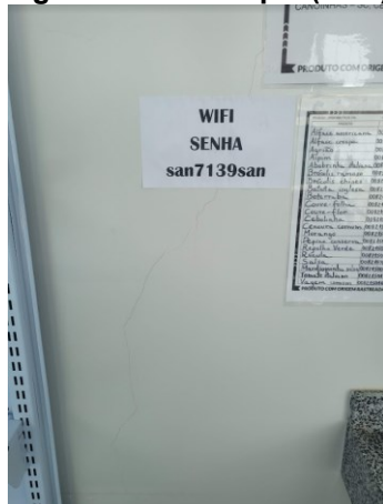
Figura 44 – Recalque (Fi=2)
