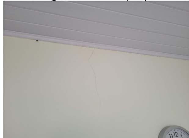
Figura 52 – Fissuras ( F_i=1 )
