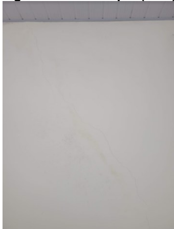
Figura 51 – Recalque ( F_i=2 )
