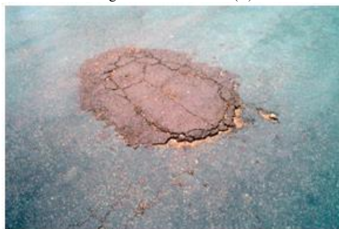
Figura 36 - Remendos (R)
