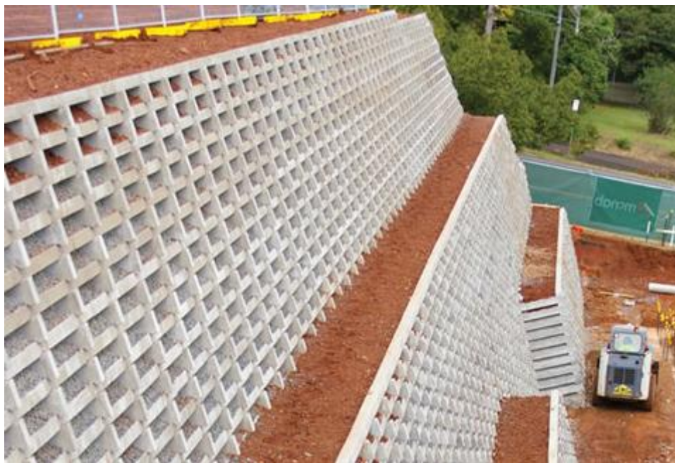
Figura 3 – Cribwall Fonte: Concrib (2014)
