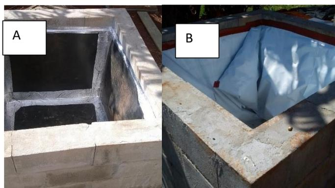
**Figura 20 – (a) Manta PEAD soldada, (b) lona dupla camada.**
